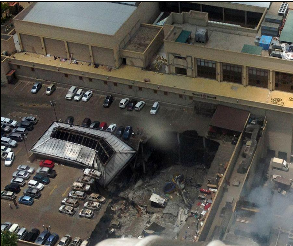
Overhead view of the collapse of the Nakumatt's rooftop parking lot
