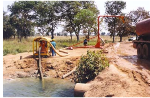
Picture 3: Potable water used by the Project
