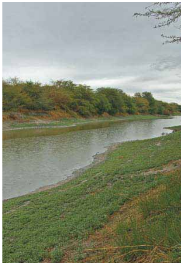
As the unfinished Jonglei canal is not connected to any major watercourse or water body, it is currently a 260 km-long ditch. The channel has been eroded and revegetated, and is seasonally flooded, supporting a new ecosystem
