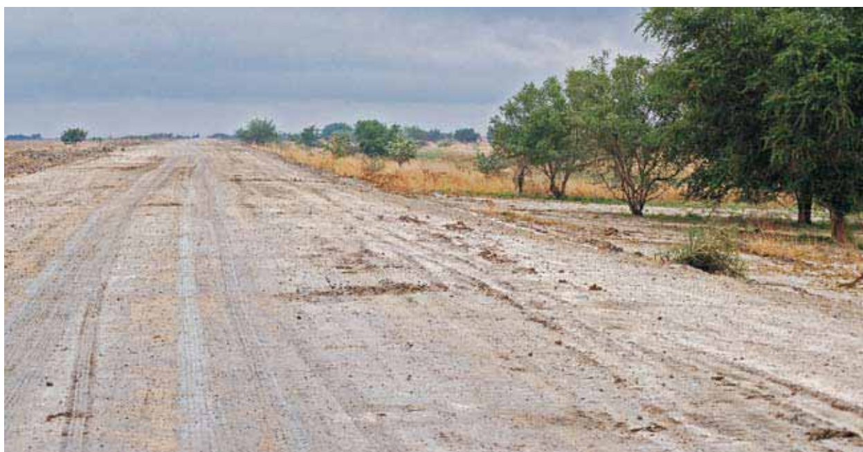
The unfinished Juba-Malakal trunk road project includes a 250 km stretch to be built on the west bank of the Jonglei canal. Approximately 100 km had been built by mid-2006, opening this remote area up for development
