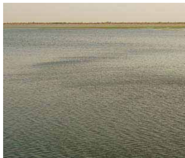
Islands and seasonal grasses are visible in the Sennar dam reservoir, which is now 60 percent full of sediment
