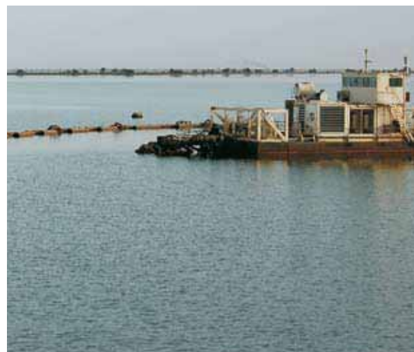
At the Roseires dam reservoir, a dredger is continuously used to remove sediment from the electric turbine water inlets. Soil washed from the Ethiopian highlands is the main source of the sediment
