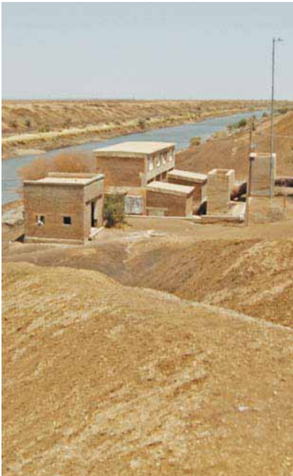
Pumping stations supply drinking water from irrigation canals that are susceptible to contamination from aerial pesticide application, such as this one in Deim el Masheihk on the Managil extension of the Gezira scheme
