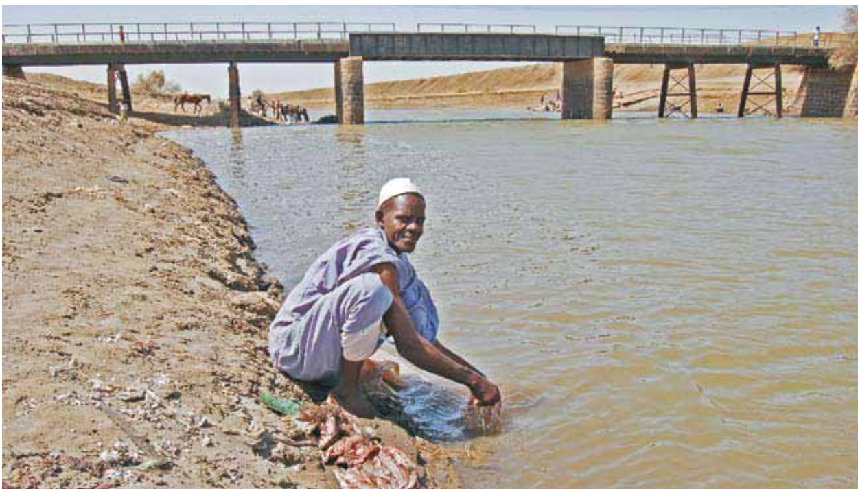
The Gezira scheme main canal and the Managil extension are used by farmers for drinking water and fishing
