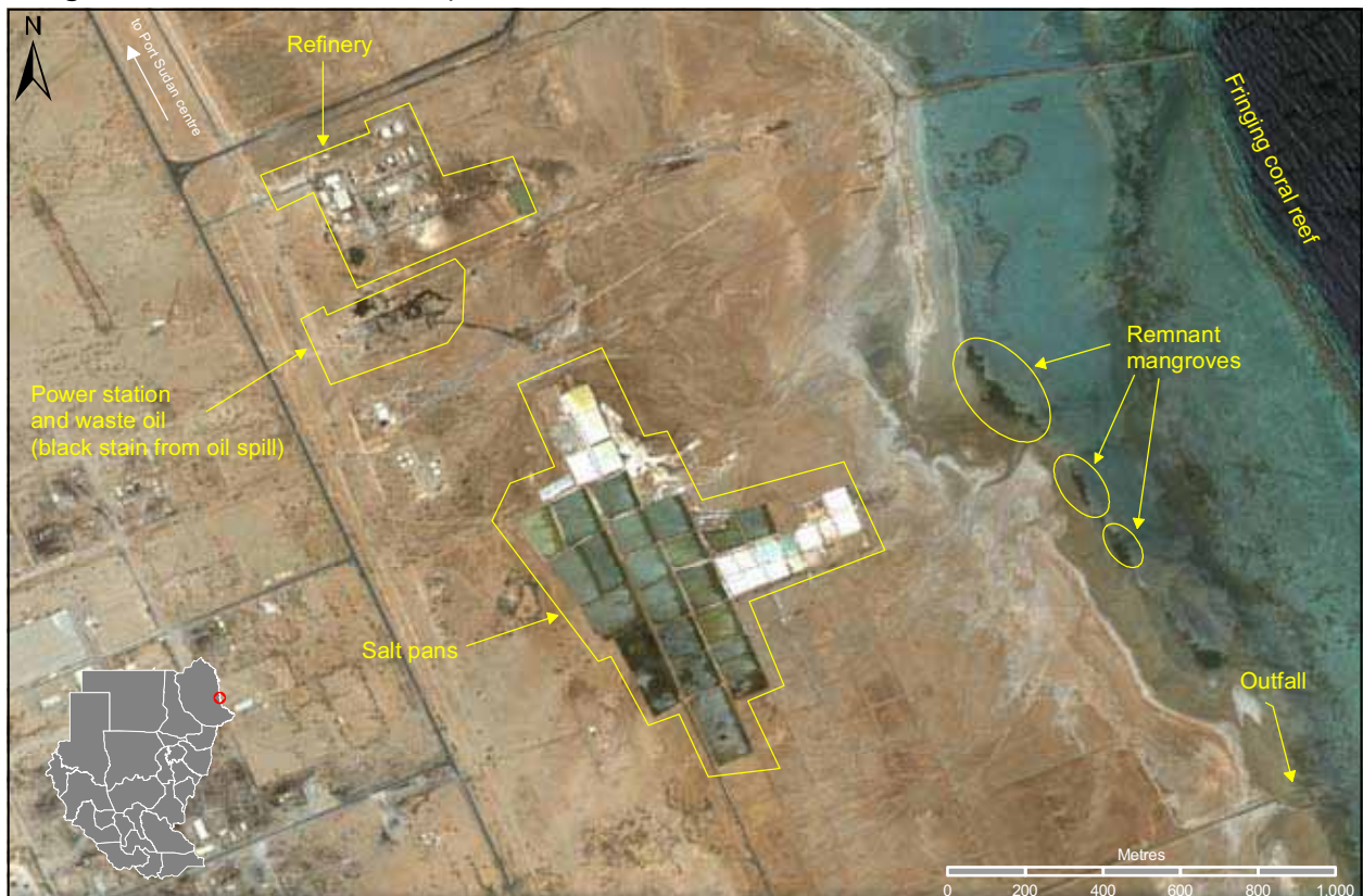
Figure 12.3 Port Sudan power station and salt flats
