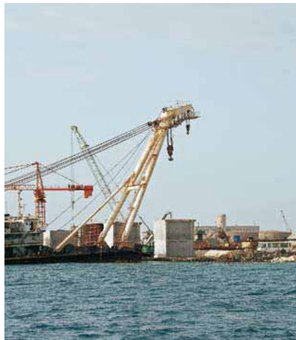
The construction of this major new harbour facility in Port Sudan proceeded without an environmental impact assessment or mitigation of its impacts
