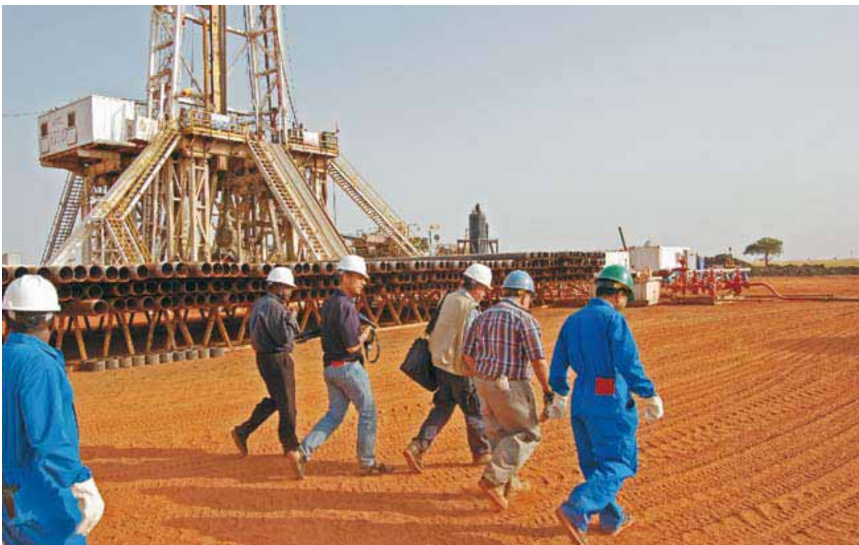
Well casings lined up beneath the Heglig drilling rig. Oil production is rapidly increasing in Sudan, as new fields are developed and transport infrastructure such as trunk pipelines and marine terminals is constructed
