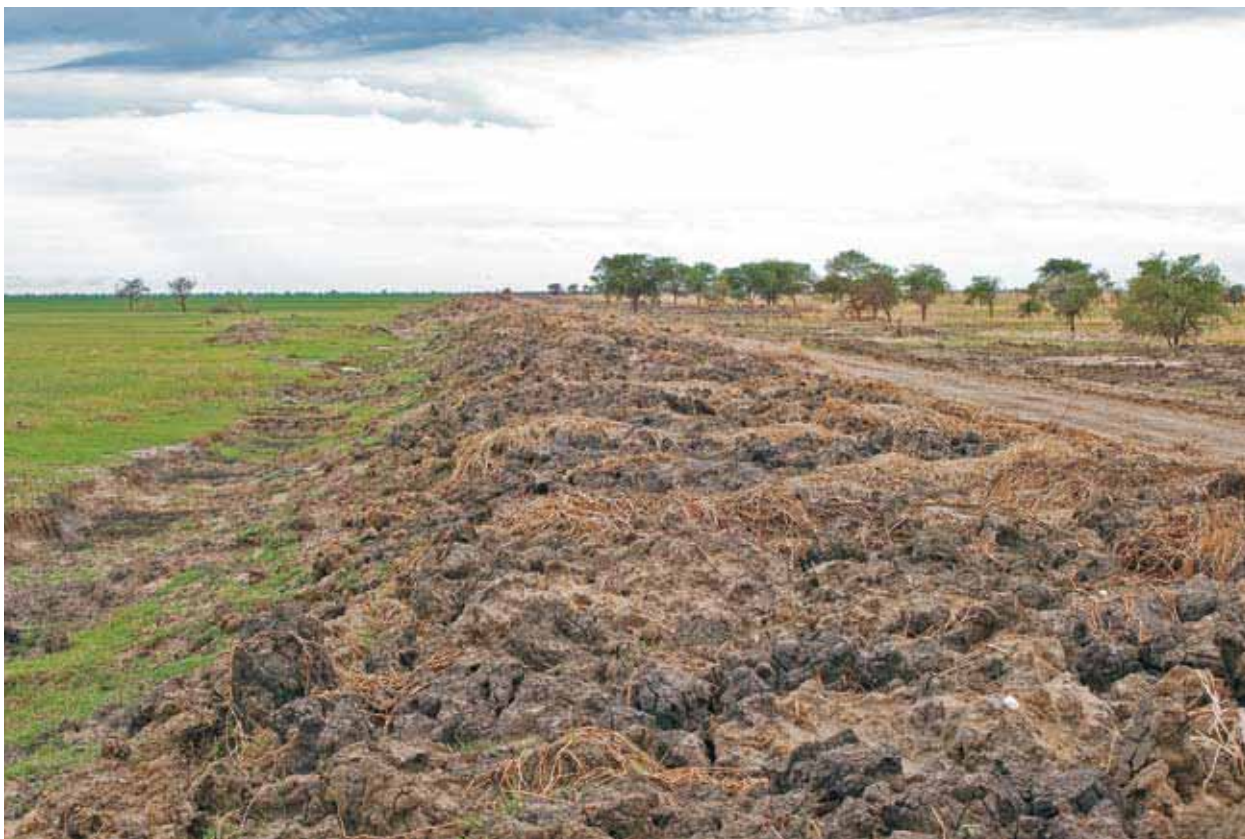
The dyke by the Bor-Padak rural trunk road was dug to control flooding in the region, but is now a cause for concern as it is leading the land beyond it to dry out and is thus reducing grazing land for both livestock and wildlife
