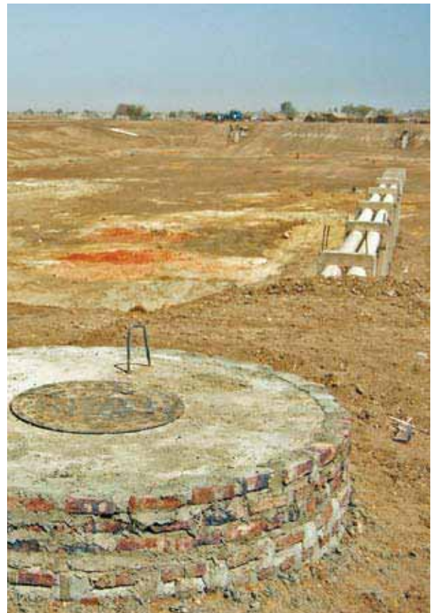
Settlement pond under construction at the Kenana Sugar Company, located near Kosti, which has recently invested heavily in the construction of water treatment facilities
