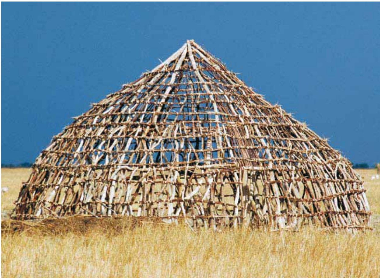
Traditional buildings such as this barn under construction near Mabior in Jonglei state require a large number of young trees
