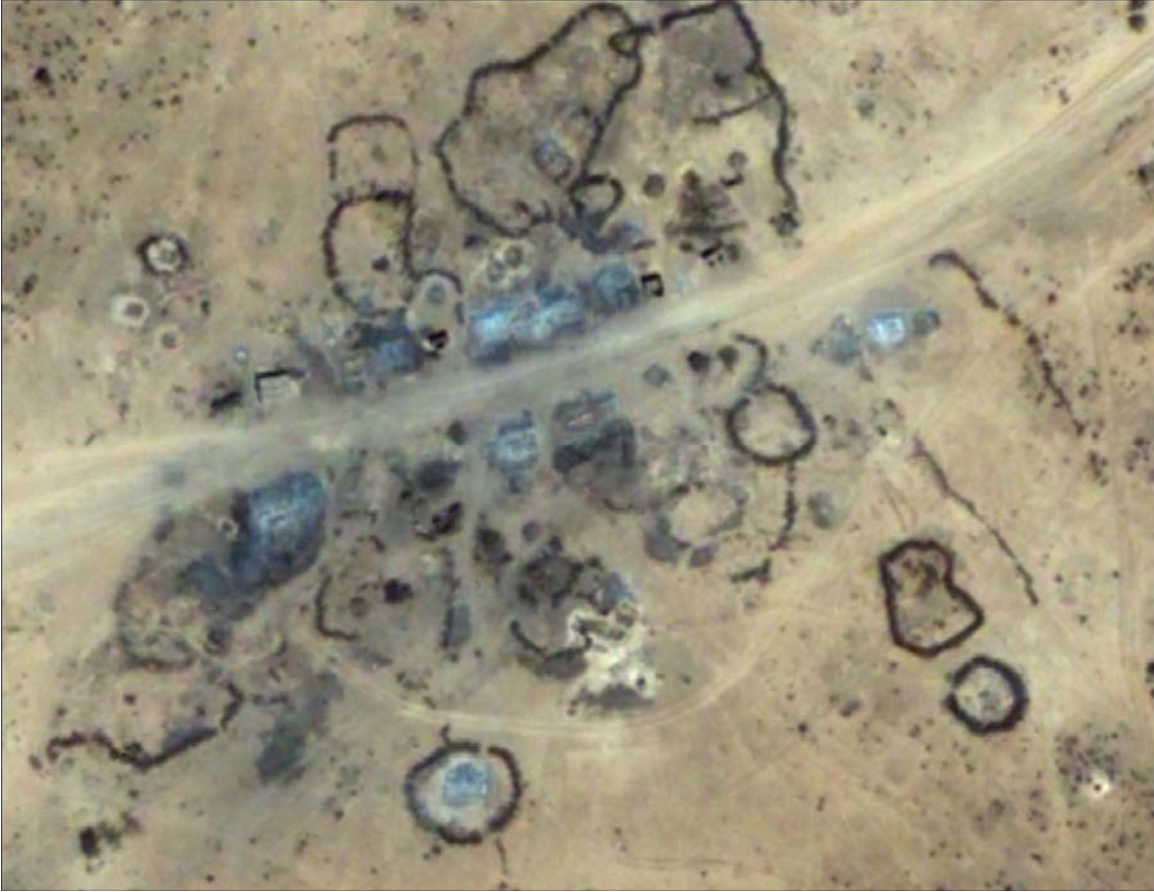
Labiga— February 28, 2008: Almost the entire town (about 40 structures) was likely removed or damaged subsequent to the collection of the previous image, and the grey/white areas are possible evidence of burning. © 2008 DigitalGlobe.
