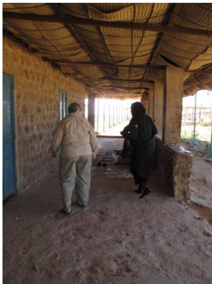
The wall in the area where interviews were conducted provided privacy when the parties were seated. (Dr. Sondra Crosby)
