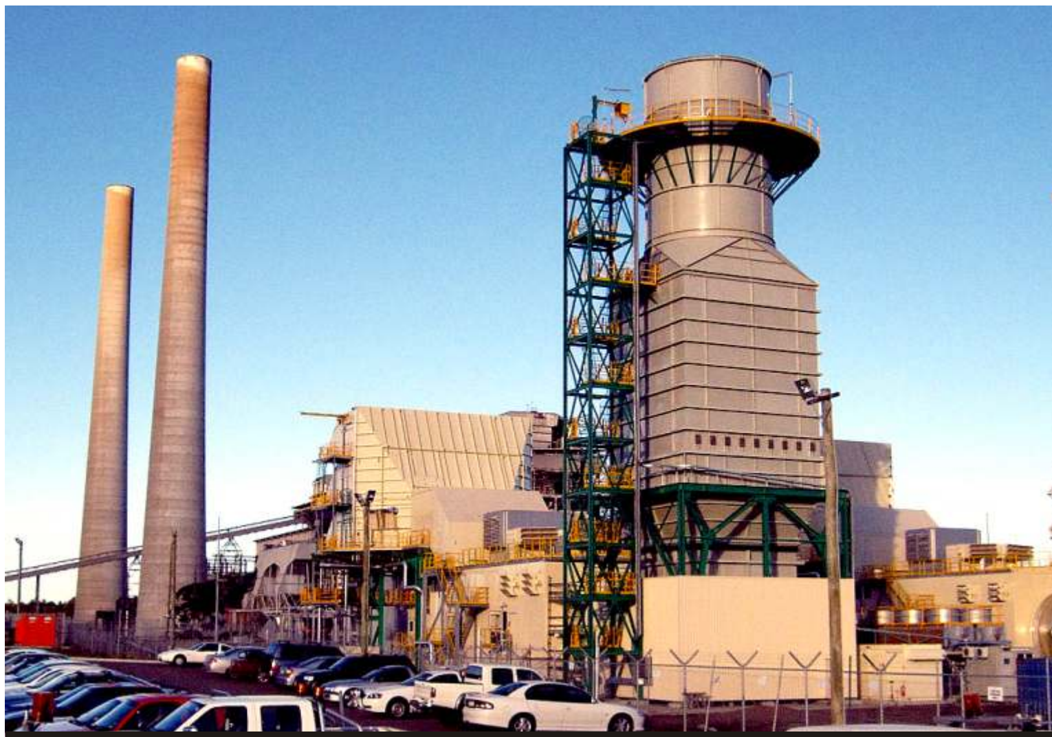
● A gas power plant
