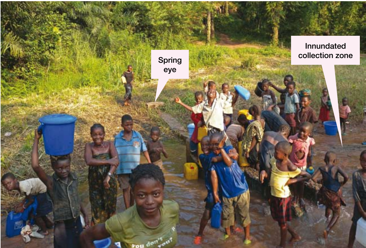
Stagnant water pools and low flow rates are indicative of poorly built spring boxes. Moubaka spring in Kikwit, Bandundu Province
