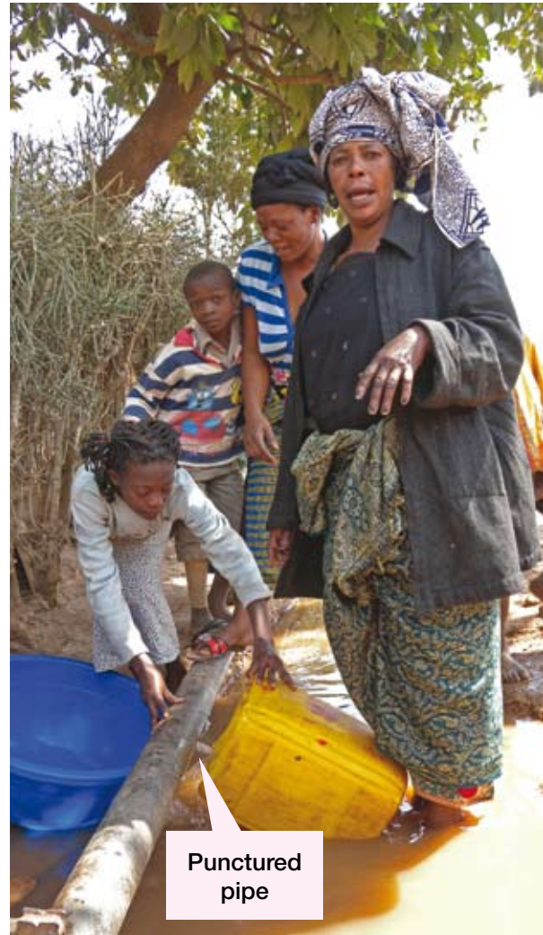
Local residents queuing in the Cité Musonoie in Kolwezi to draw water from breaches in the water pipeline (Katanga Province)
