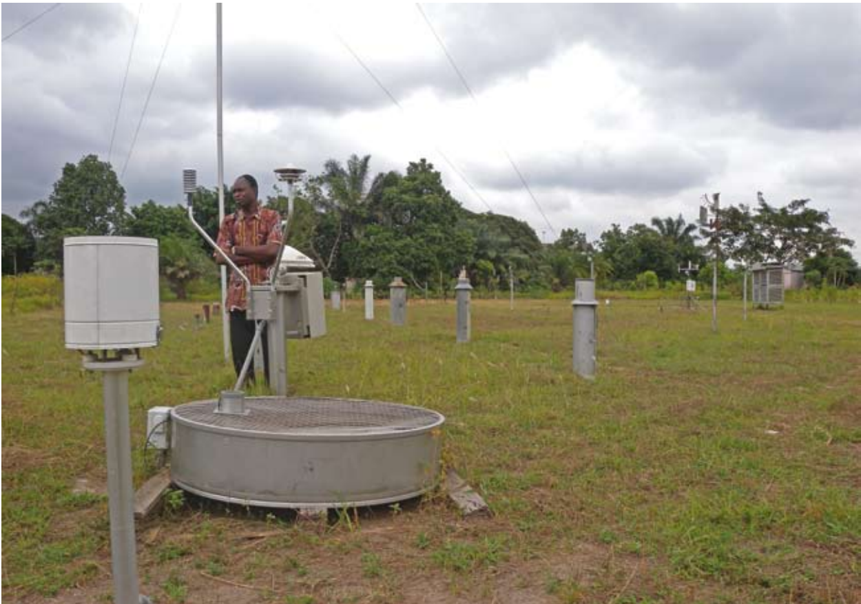
To rehabilitate its collapsed weather monitoring network, METTELSAT recently installed automated weather stations
