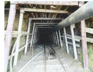
Tunnel under construction
