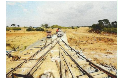
Rail line into the tunnel under construction
