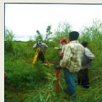
Laying of Baseline Survey Points
