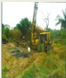
Diamond core drilling in progress
