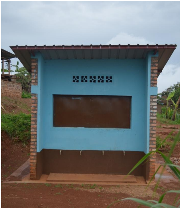
FIGURE 3-5 COMMUNITY DRINKING WATER TAP IN MUYEBE VILLAGE
