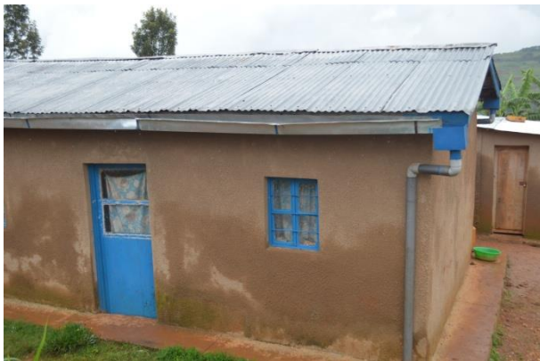
FIGURE 3-2 ROOFTOP RAINWATER HARVESTING
