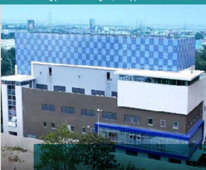
District cooling plant in Northgate, Philippines
