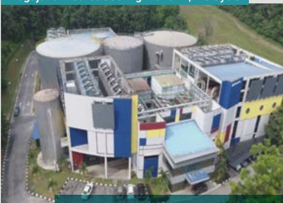
Megajana District Cooling Plant #1, Malaysia
